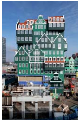
2. westgevel/ west facade
